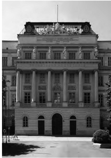
Figure 3-2 Original Building on Karlsplatz
