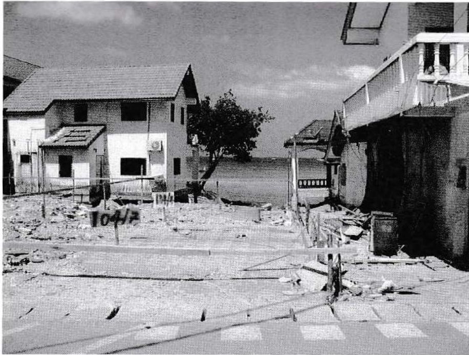
Figure 2: Kamala beach, showing a destroyed building, now just a plot of land.
